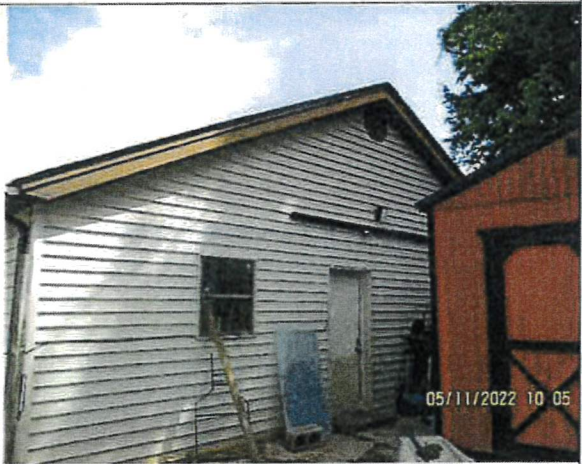
EXTERIOR SIDE C
